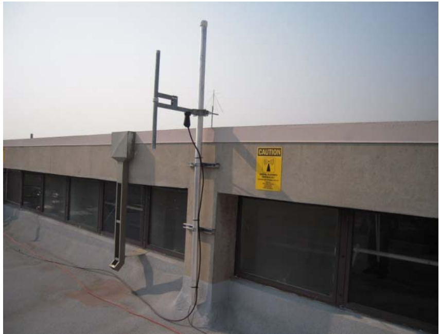
Figure 2. Interoperability communications laboratory roof-mounted antenna with caution sign located next to the antenna.
